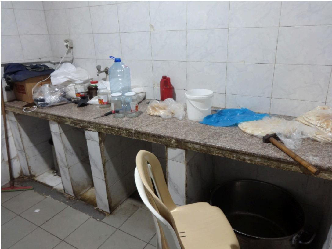
The countertop in the main kitchen in Tripoli Men's Prison
